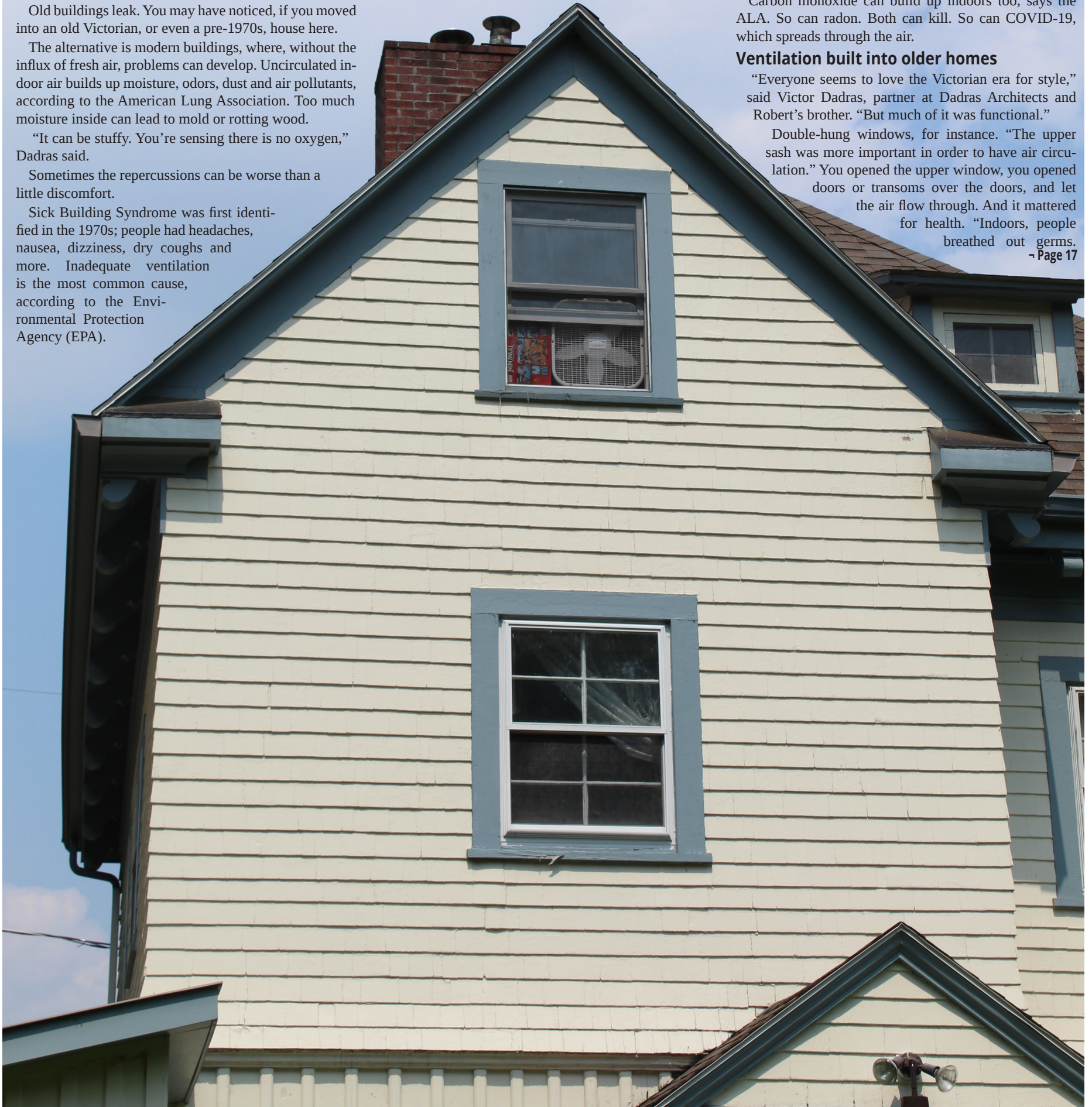
This is an easy way to ventilate a hot attic: an open window and a box fan to blow air in or out of the room.
