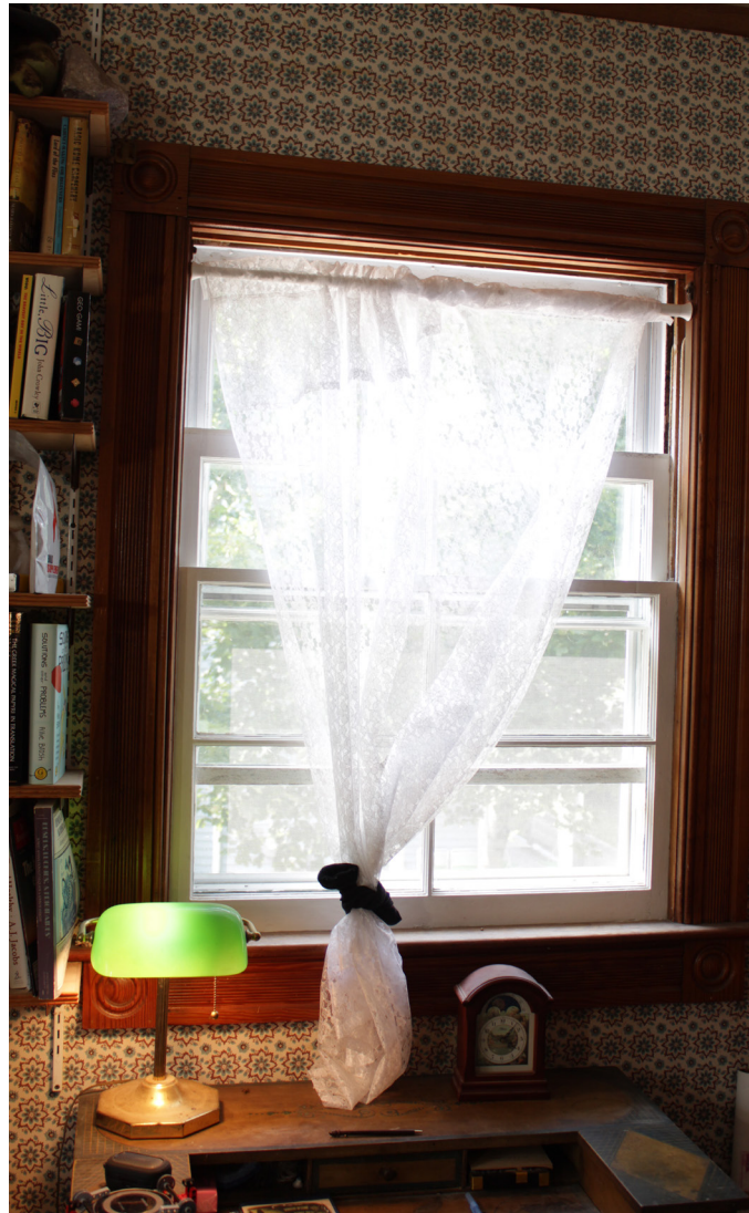
RR photo by Joe Cooke A double-hung window, ventilating.
